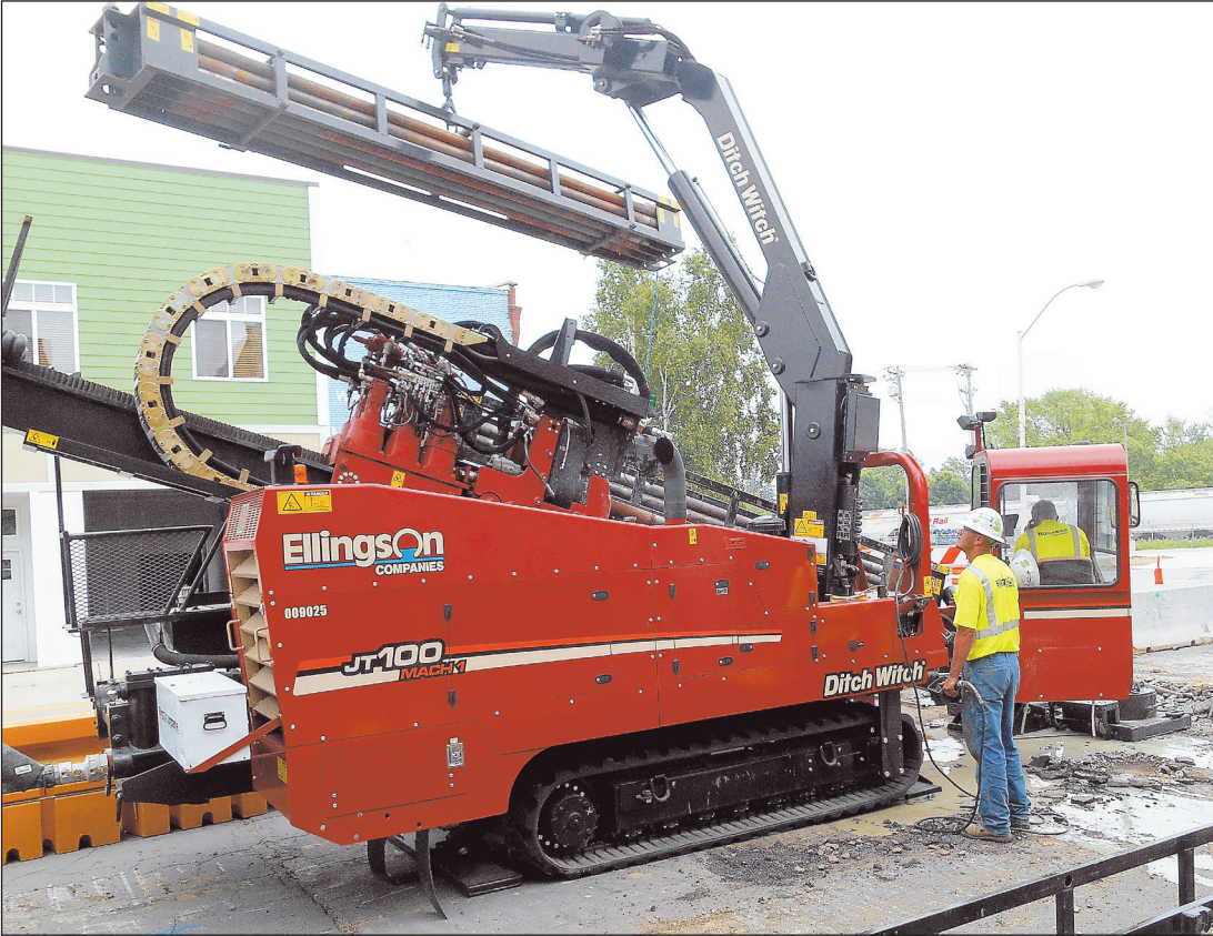
Staff file photo by Howard Lestrud Ellingson Companies of West Concord last week started some directional drilling on the Main Street reconstruction project in Blooming Prairie. The drilling was done to place utilities underground. Initial street construction across 218, east to 5th Ave. included removal of pavement and curbing.
