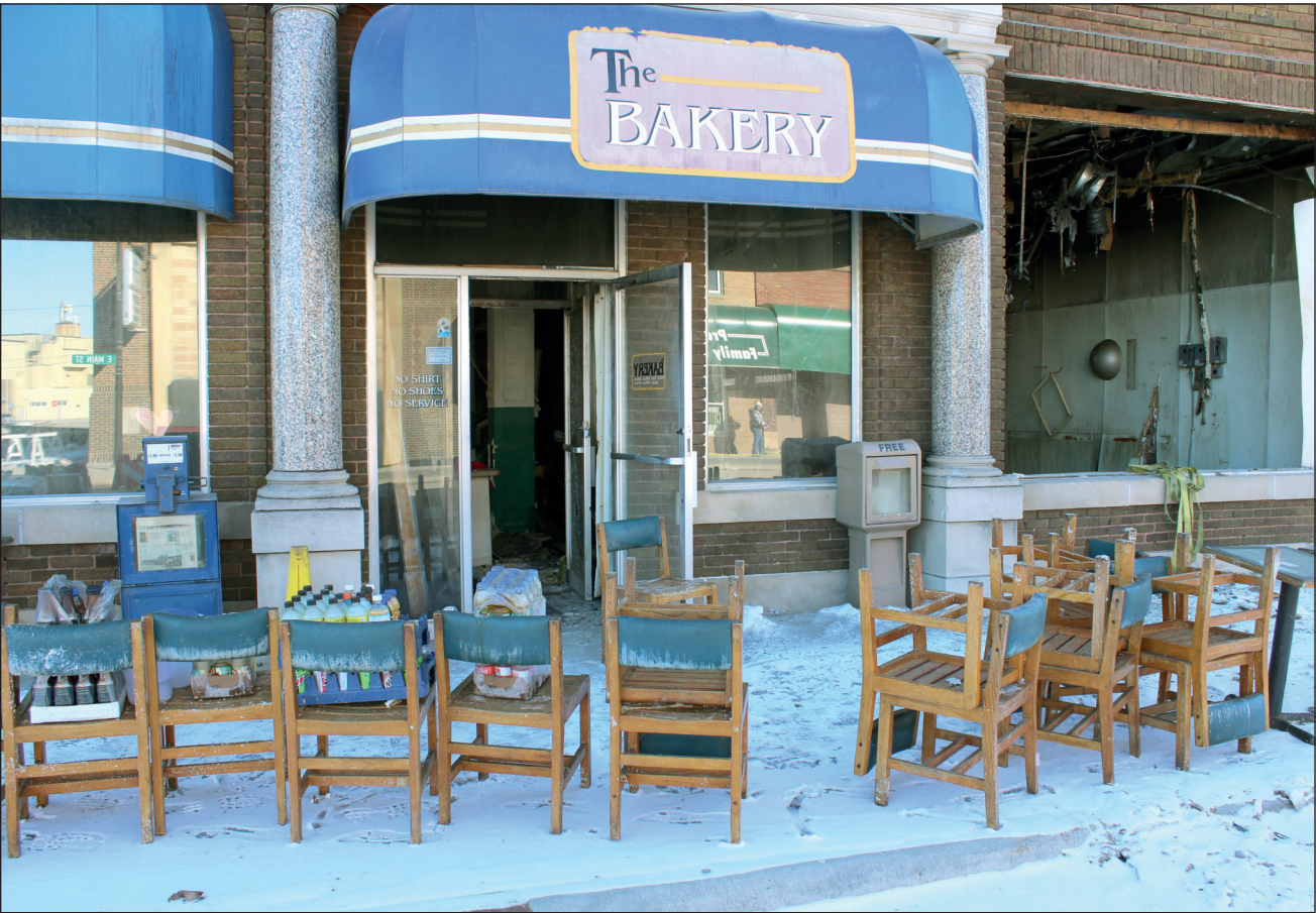
Now, the salvage begins at The Bakery. Insurance and State Fire Marshal investigators have been on the site of The Bakery and Sportstitch on many occasions since the Jan. 28 fire.
