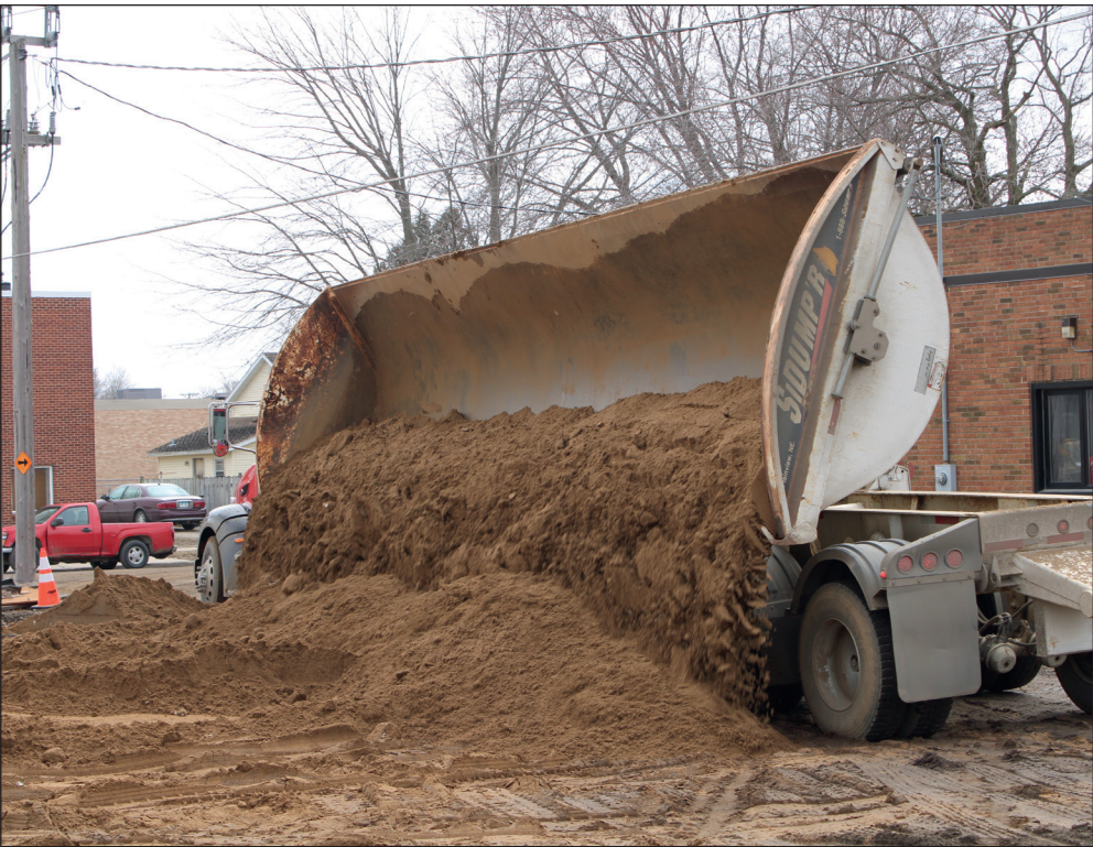
More fill was brought to the site of The Bakery. Keith Johnson, owner of KJ Construction Co., said 150 loads of dirt were brought to the site of The Bakery and Sportstitch.
