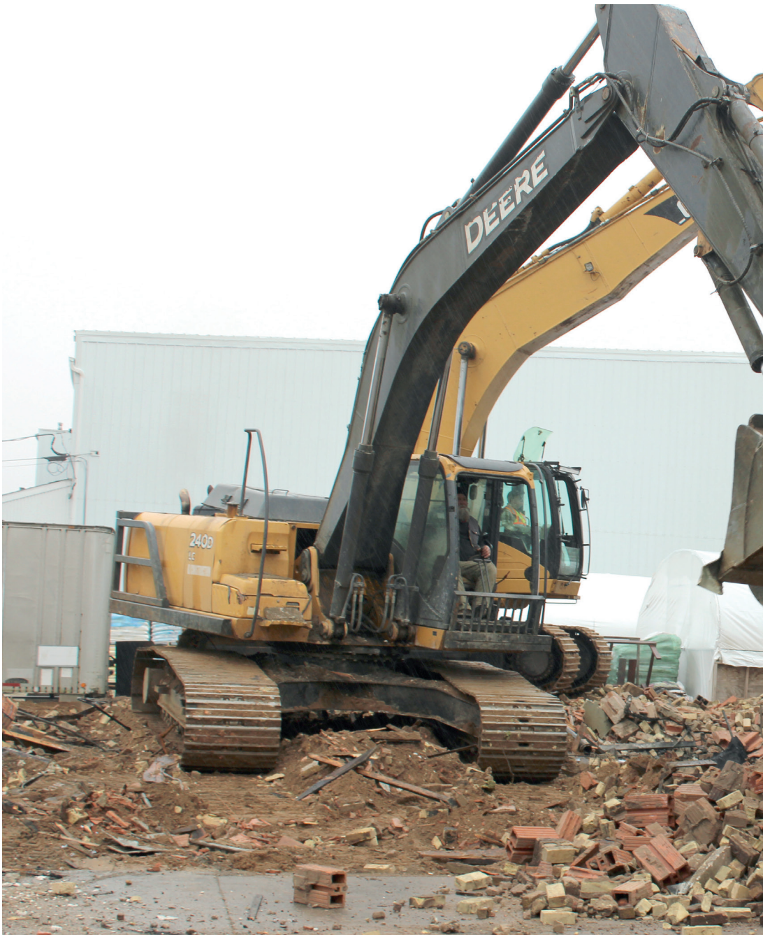
At times, it looked like demolition on Blooming Prairie's Main Street was an act of double vision. Here, two
