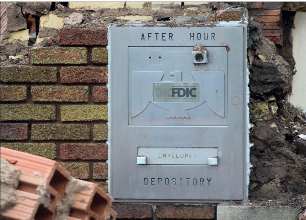
A night deposit from the old First National Bank of Blooming Prairie was uncovered by KJ Construction Company during demolition work last week.
