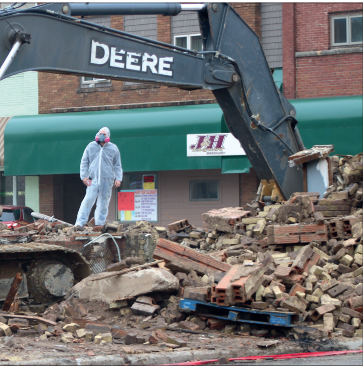
last week, searching for asbestos in the walls of The Bakery building.
