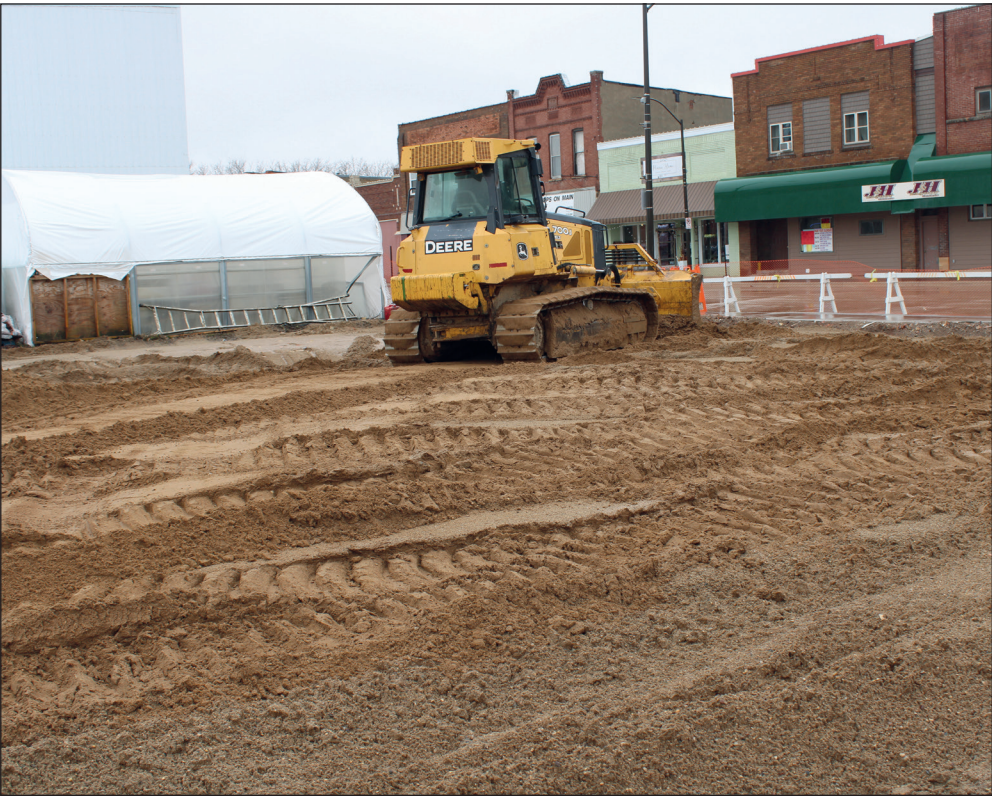
After filling in the site of The Bakery, Keith Johnson of KJ Construction said the work is finished except for a layer of black dirt to be placed over the sand fill. The project began on March 18 and was to be completed by April 3.
