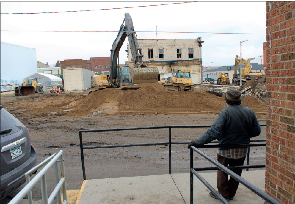
Howard Hill spent lots of hours watching the demolition of The Bakery and Sportstitch. He chronicled the project with his trusty digital camera.
