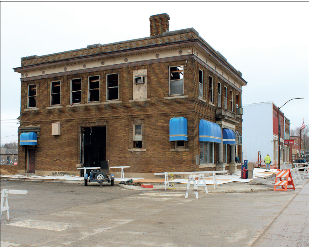
The old First National Bank building, which also became the home of The Bakery, stands tall before it was taken down by demolition experts last week.
