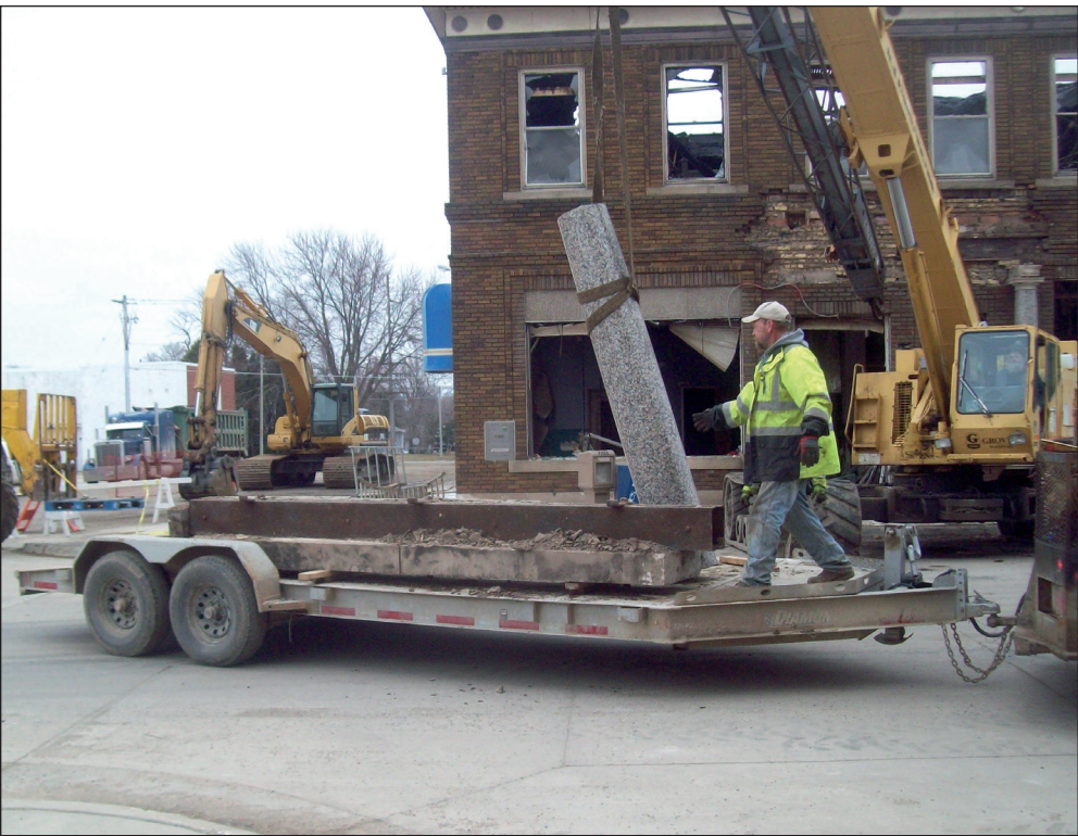
Two granite pillars on the front side of The Bakery building were salvaged in excellent condition.
