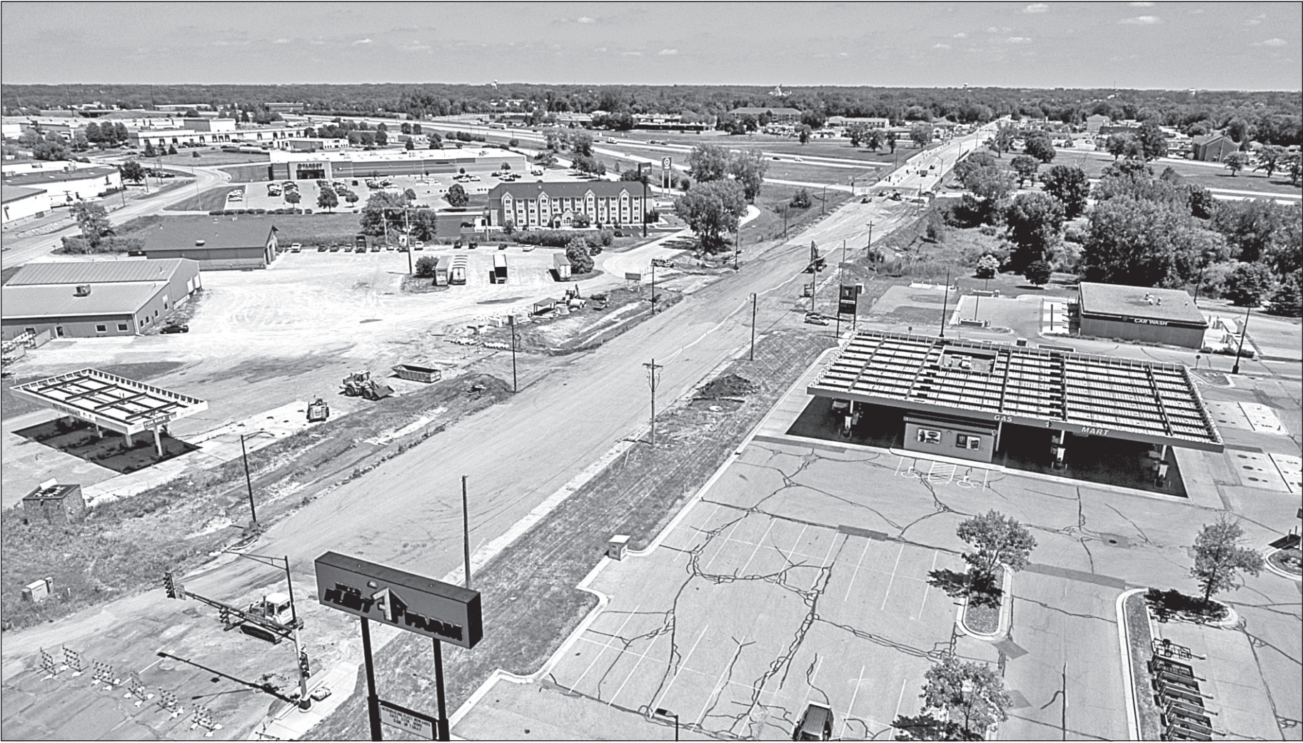
As reconstruction of Bridge Street from I-35 to 24th Avenue continues, this aerial drone shot shows the aggregate road base and work along the north road ditch. Phase 1 work began on May 1 and all work is scheduled to be substantially complete no later than Oct. 30.
