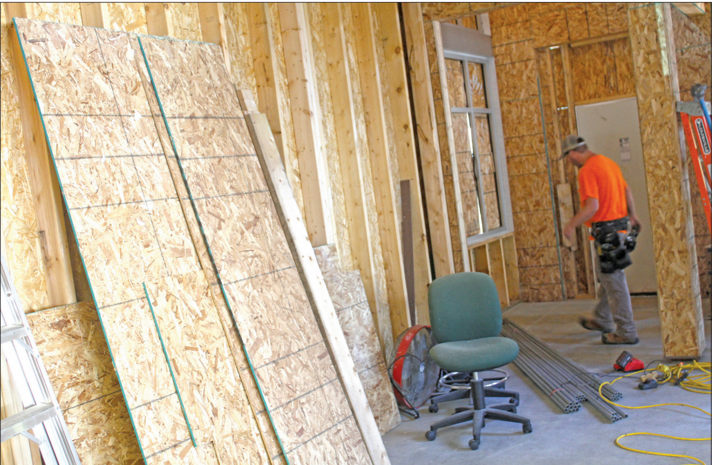
Construction of the new all in one Home Federal building in Kasson is continuing to stay on progress, despite the inclement weather we have been experiencing this summer. The bank hopes to move into the new building by the end of September.
