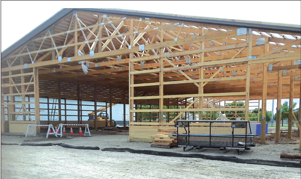
The new cattle barn being constructed on the Steele County Fairgrounds in Owatonna. This new barn will be replacing two older barns, one of which had its roof damaged in the winter. The barn is to be named after the Kubiceks: Wayne and Betty Kubicek Family Cattle Haven.
