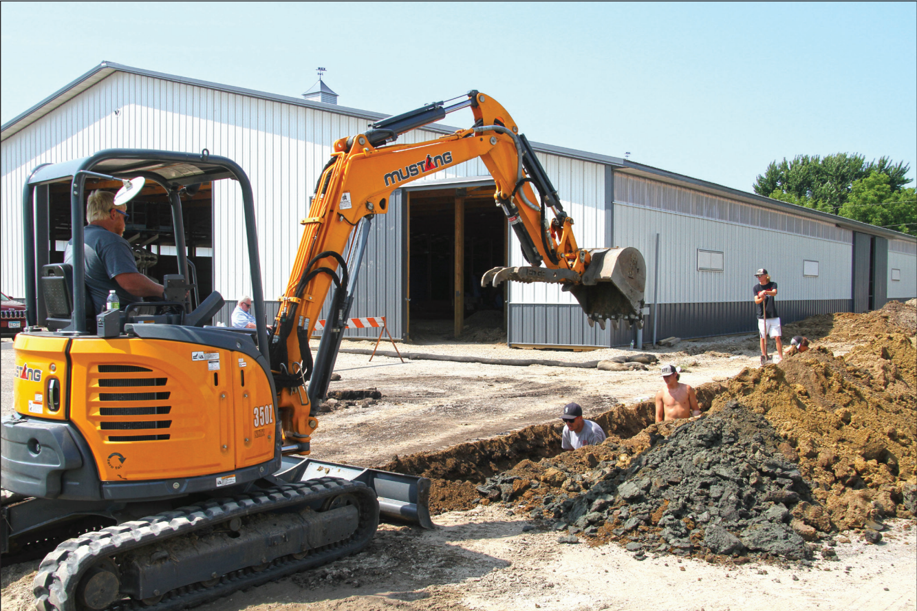
STAFF PHOTO BY RICK BUSSLER The grounds crew at the Steele County Free Fair in Owatonna keeps busy getting the new barn ready for the fair. With the aide of a back hoe, crew members last week dug a trench in an effort to install a water line for the new wash rack located on the side of the barn. Fair manager Scott Kozelka says the barn will be complete and ready for dairy animals in time for the fair, which begins on Aug. 13 and runs until Aug. 18. The barn is just one of several major projects on the grounds this summer.
