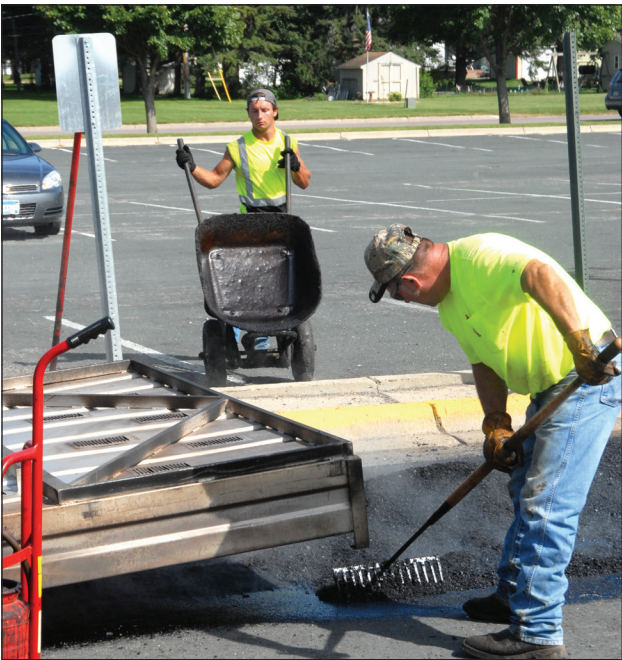
Workers of this Mountain Lake business firm apply some blacktop patches on the street by the Blooming Prairie High School to get ready for the first day of school on Sept. 3.
