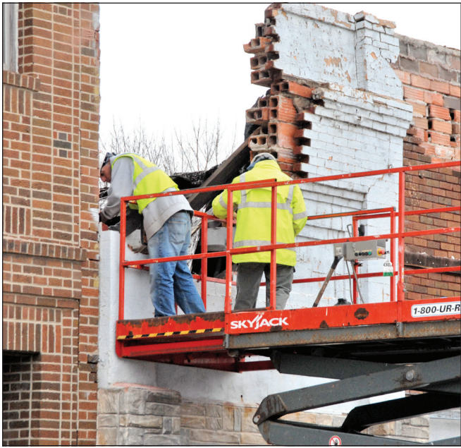
STAFF PHOTO BY HOWARD LESTRUD The Blue Earth Environmental Co. of Mankato last week began demolition of the old Hansen Building, located at 108 3rd Ave. NE.
