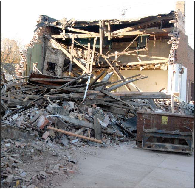
STAFF PHOTO BY HOWARD LESTRUD Workmen last week were busy demolishing the old Hansen Building, located at 108 3rd Ave. NE in Blooming Prairie. The building once housed a movie theatre.
