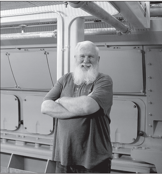
From Blooming Prairie to booming engines, project manager Todd Manchin stands next to one of the huge G20CM34 generator sets. These will be able to provide quicker, more reliable, and more efficient energy to the region.
