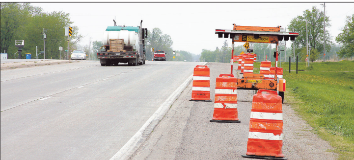
Staff photo by Alan Van Ormer Old Highway 14 construction will start soon in Owatonna.
