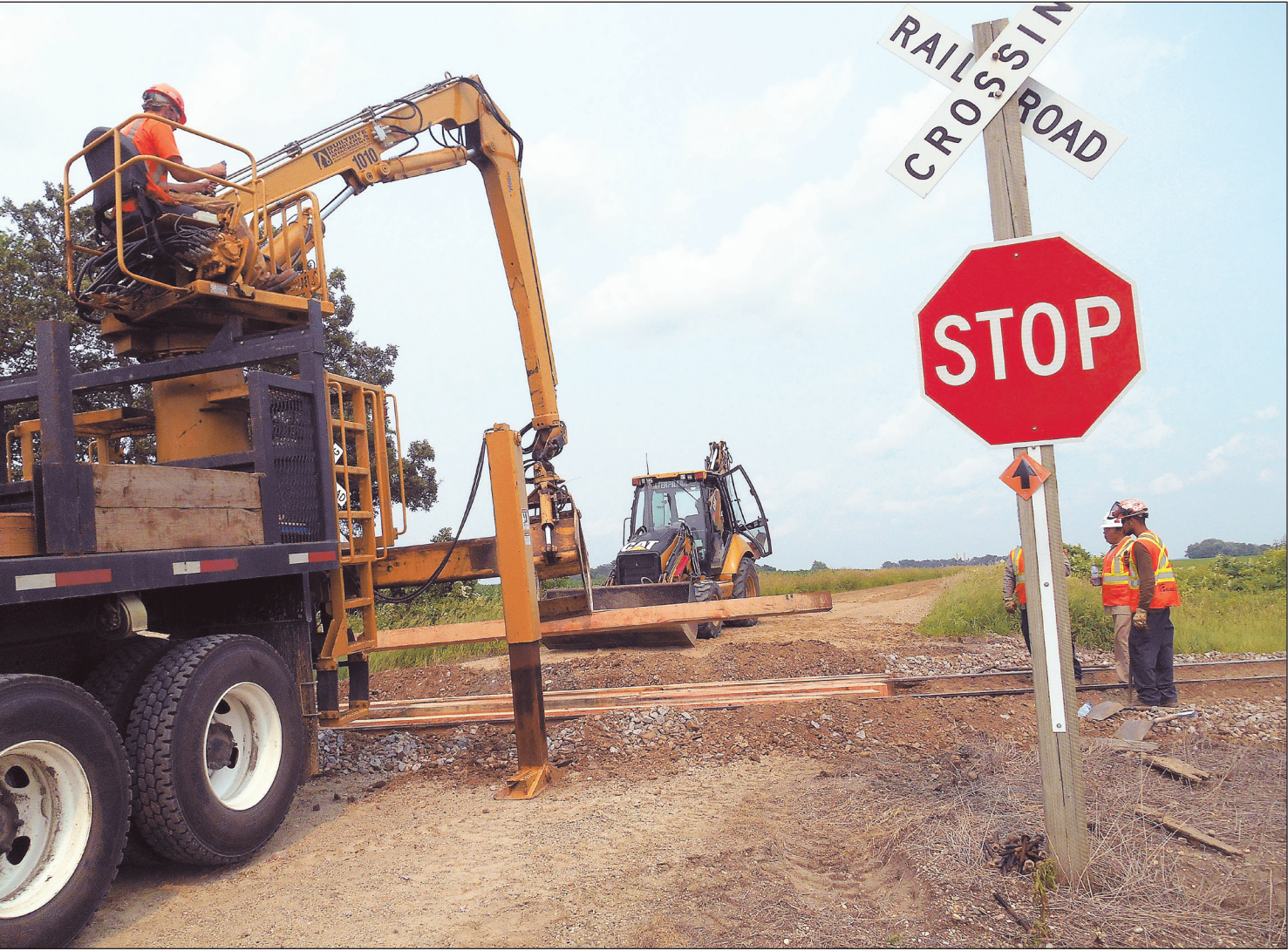
Canadian Pacific Railroad was busy lifting railroad ties and replacing them with new wooden ties in the Blooming Prairie area last week. Here, Railwork of Minooka, Illinois replaces old rail ties removed by R.J. Corman Company of Nicholasville, Kentucky. A railroad tie is a rectangular support for the rails in railroad tracks. The ties are generally laid perpendicular to the rails, ties transfer loads to the track ballast and subgrade, hold the rails upright and keep them spaced to the correct gauge.
