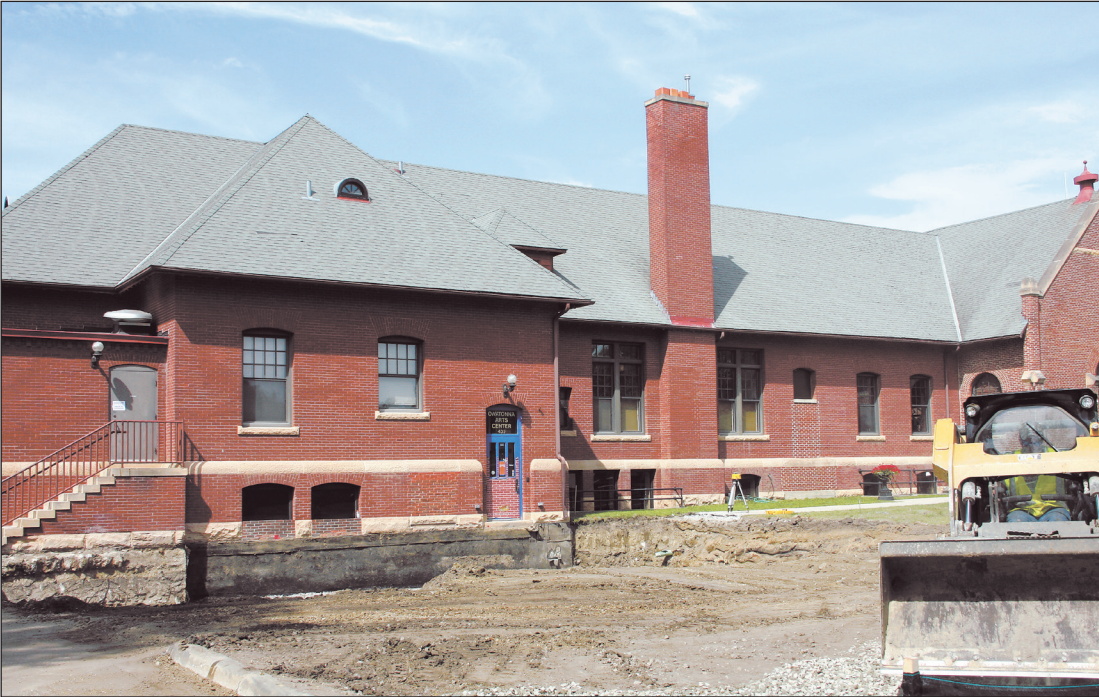
Staff photo by Anna Segner The Owatonna Arts Center is stretching out. Construction for the addition has begun to the south of the current Arts Center and will include a handicapped accessible entrance and a bit more gallery space.
